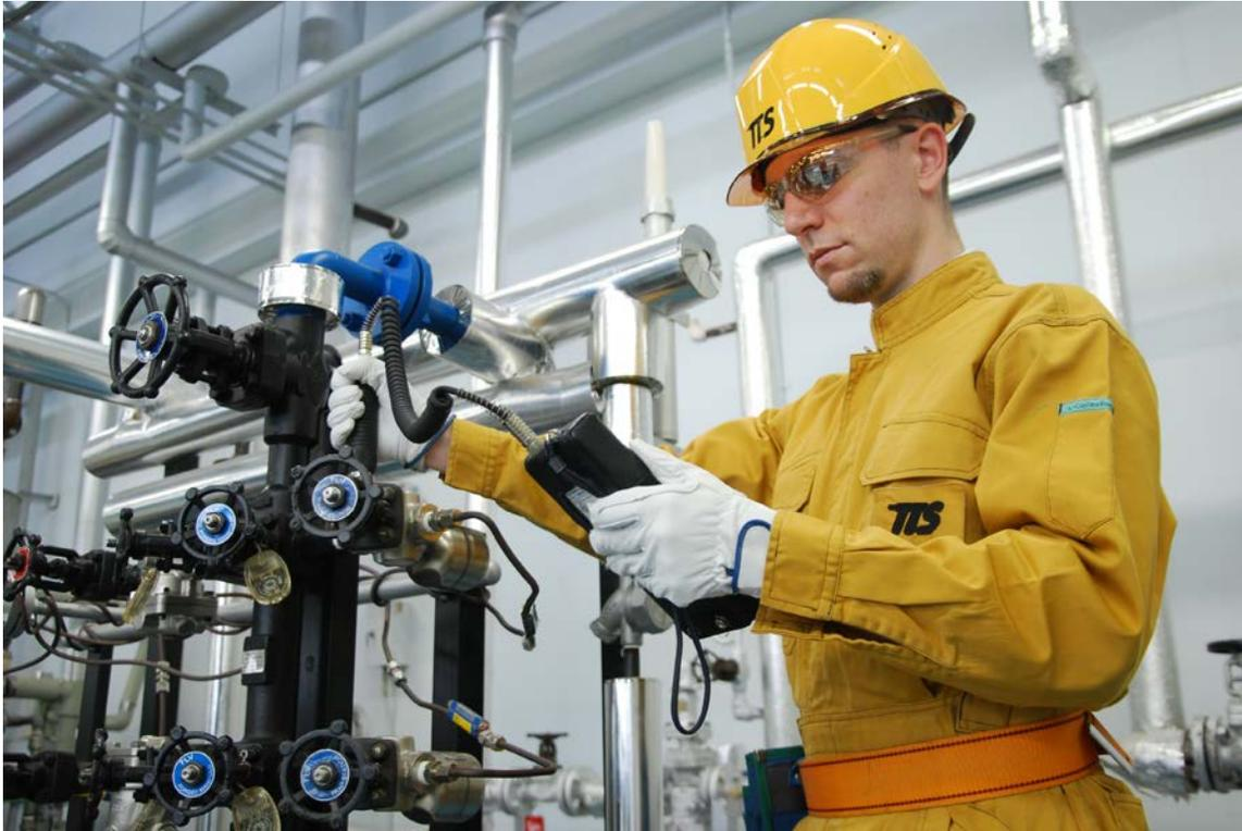
**Figure 3: A steam trap survey is an essential component of a steam trap management program. TTS Photo courtesy of TLV Co., Ltd.**
