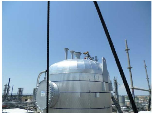
**Figure 2. Top head of a distillation column after applying insulation (left) and after securing jacketing (right). Courtesy Aspen Aerogels, Inc.**
